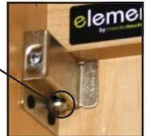
Raising the cabinet to the highest point eliminates the space required to lift the cabinet enough to remove the lip of the clip from the track.
